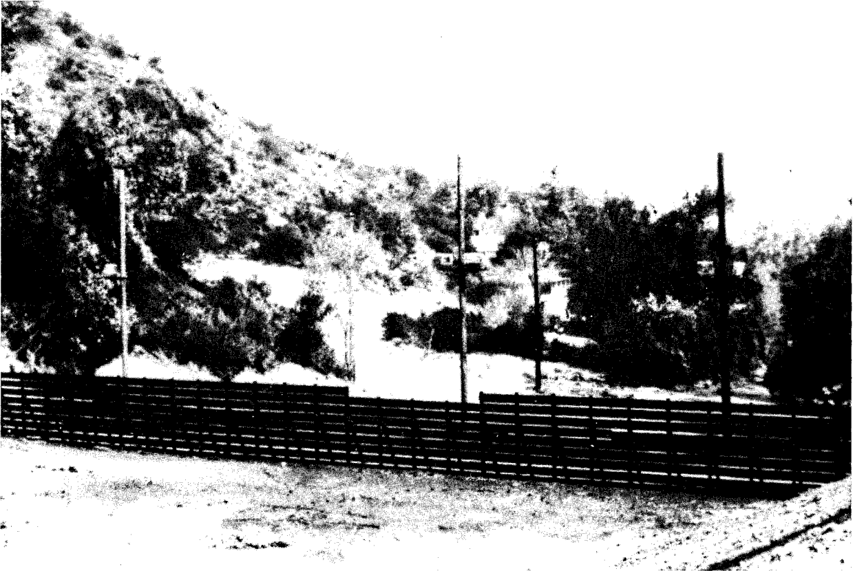
Emergency Fire Structure - Serving to Protect Downstream Development from Debris Flows
